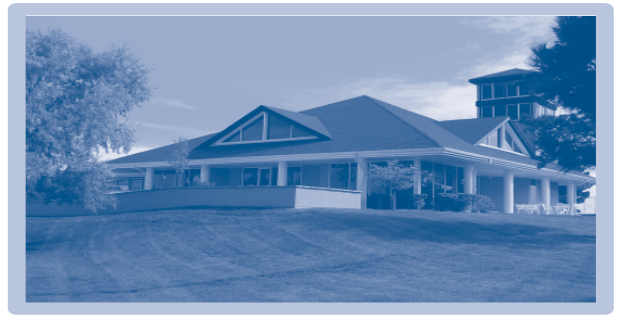
Castle Pines North Metro District Building
