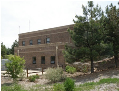
CPNMD Water Treatment Plant
